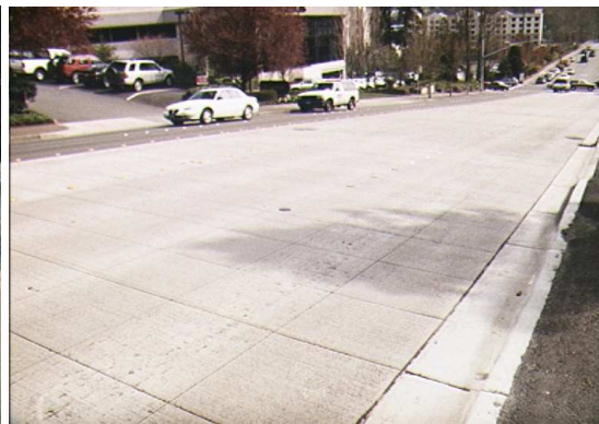
Figure 2. Completed pavement and curb detail, looking eastbound.
