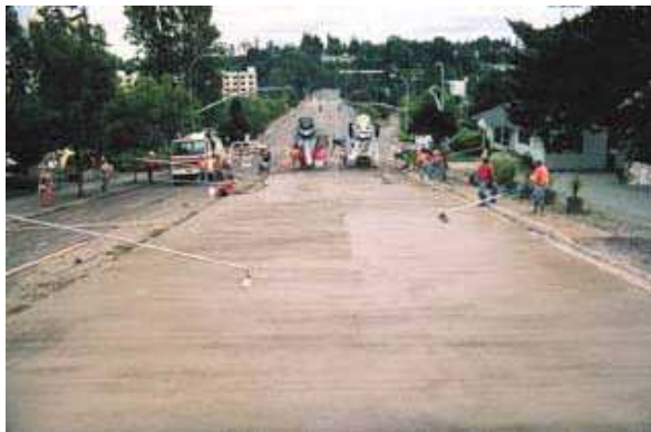
Figure 1. During construction, looking eastbound.
